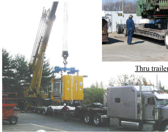
Machinery delivered, uncrated and set in place
